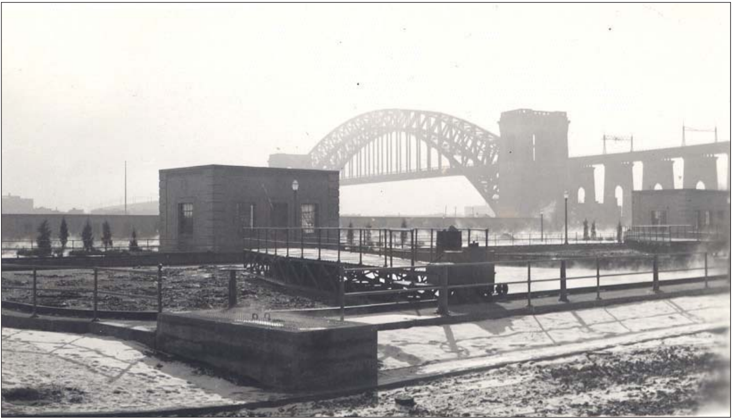
Wards Island Wastewater Treatment Plant - 1938
